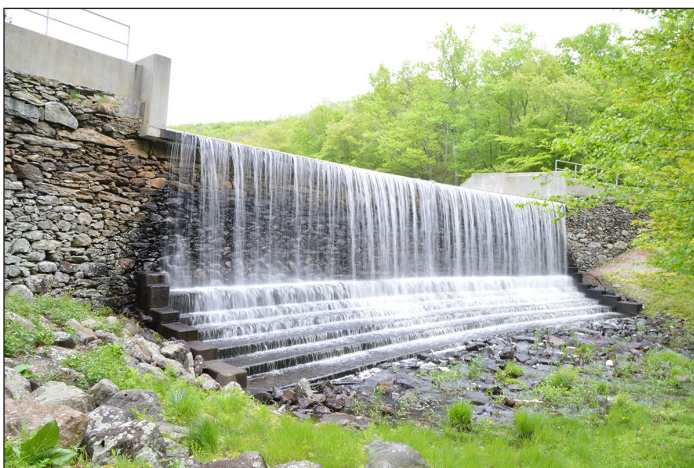
Deep Hollow Reservoir Dam
